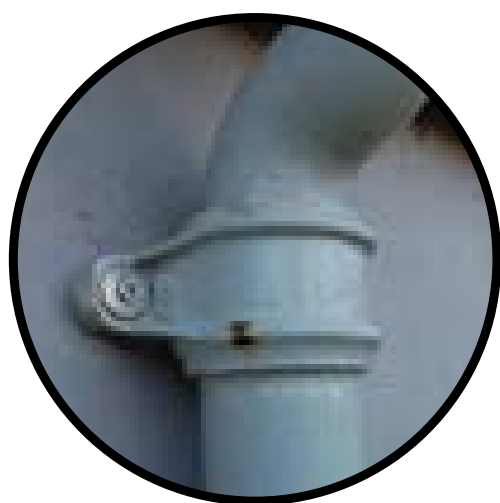
Examples of chips and scuffs after installation painting that have not been re-touched, resulting in rusting of damaged area
