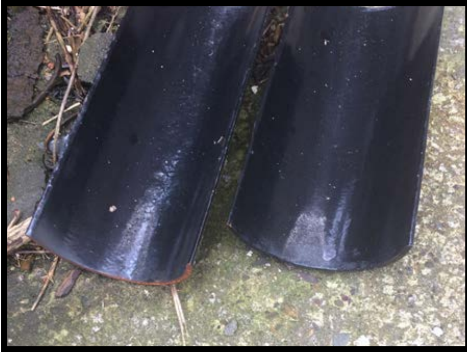
PX Painted Gutter
