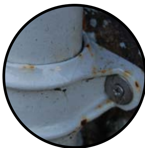
Examples of chips and scuffs after installation painting that have not been re-touched, resulting in rusting of damaged area
