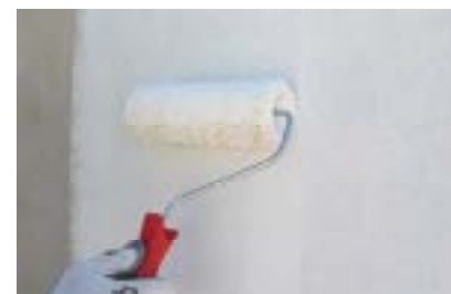
17. Application of SecilTEK SP 01 on SecilTEK AD 25
