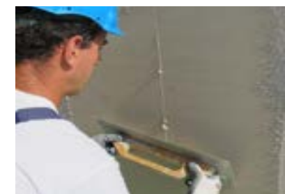
14. Application of first layer of REABILITA Cal Acabamento (Finish)
