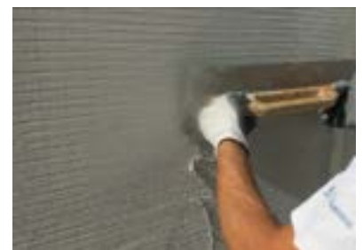
13. Second spreading of ADHERE Vit ecoCORK
