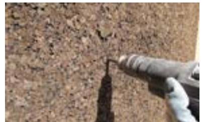
7. Drilling holes for putting mechanical fixing
