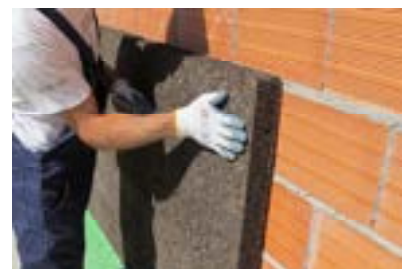
4. Fixing the panel by pressing it
