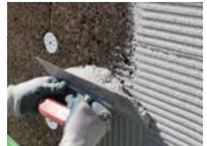
11. First spreading of ADHERE Vit ecoCORK
