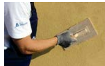
19. Application of acrylic finish REVDUR
