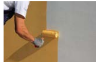
18. Application of primer SecilTEK AD 20
