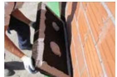
3. Placing the panel on the support
