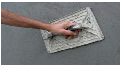
Trowelling the final surface
