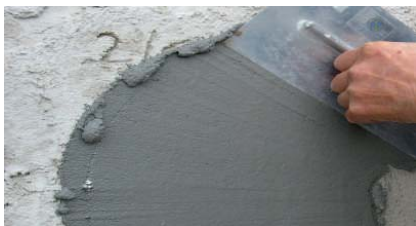
Execution of first layer
