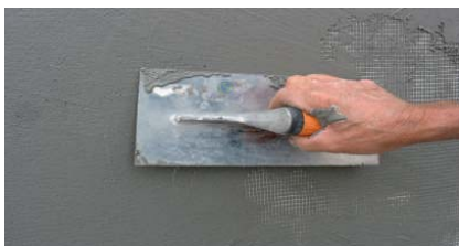
Application of the second layer
