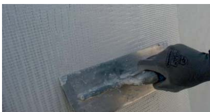
Embedding the reinforcement net
