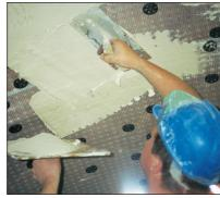
Plasters and renders should be trowel applied in two coats. The first coat of approximately 7mm is pushed into the mesh and allowed to dry, before the second coat is applied. Skim finish plaster can be used in the normal way.
