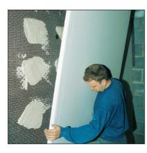
When dab fixing plasterboard the adhesive dabs are applied directly over the fixing heads. The adhesive dabs should cover 50% of the area. The boards are then wedged at the bottom and offered up to the dabs.
