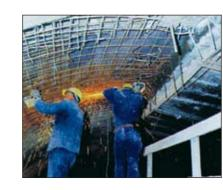
In the Brachbach tunnel project. DELTA '-PT was installed over a quickdrying shotcrete levelling layer to provide full-surface drainage.
