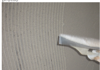
First layer over insulating boards
