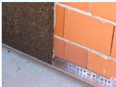
Cork panel application with startup profile
