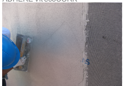
Execution of the second levelling layer of ADHERE Vit ecoCORK
