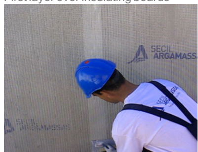
Embedding fiber glass net over ADHERE Vit ecoCORK
